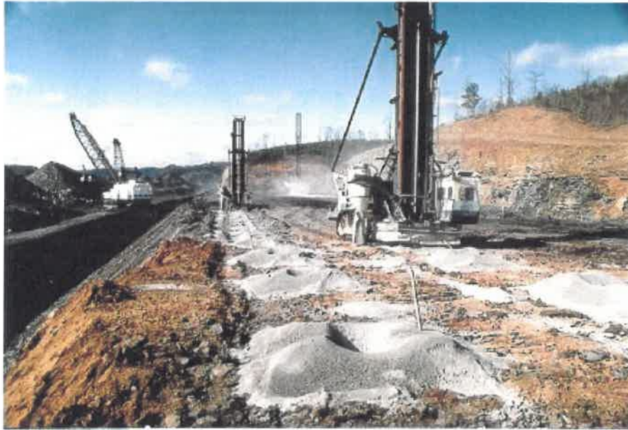
Figure 2 – Blast pattern with drill holes and drill rigs (U.S. DOI, 2023)
